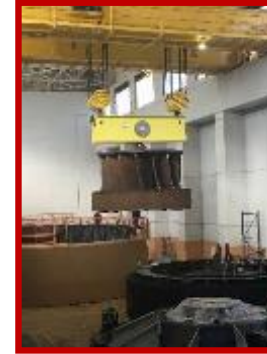
Denison Dam Turbine
